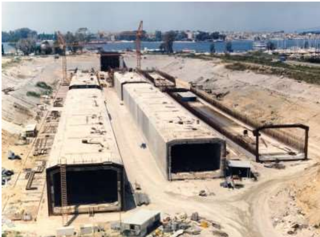
Tunnel elements under construction prior to launching
