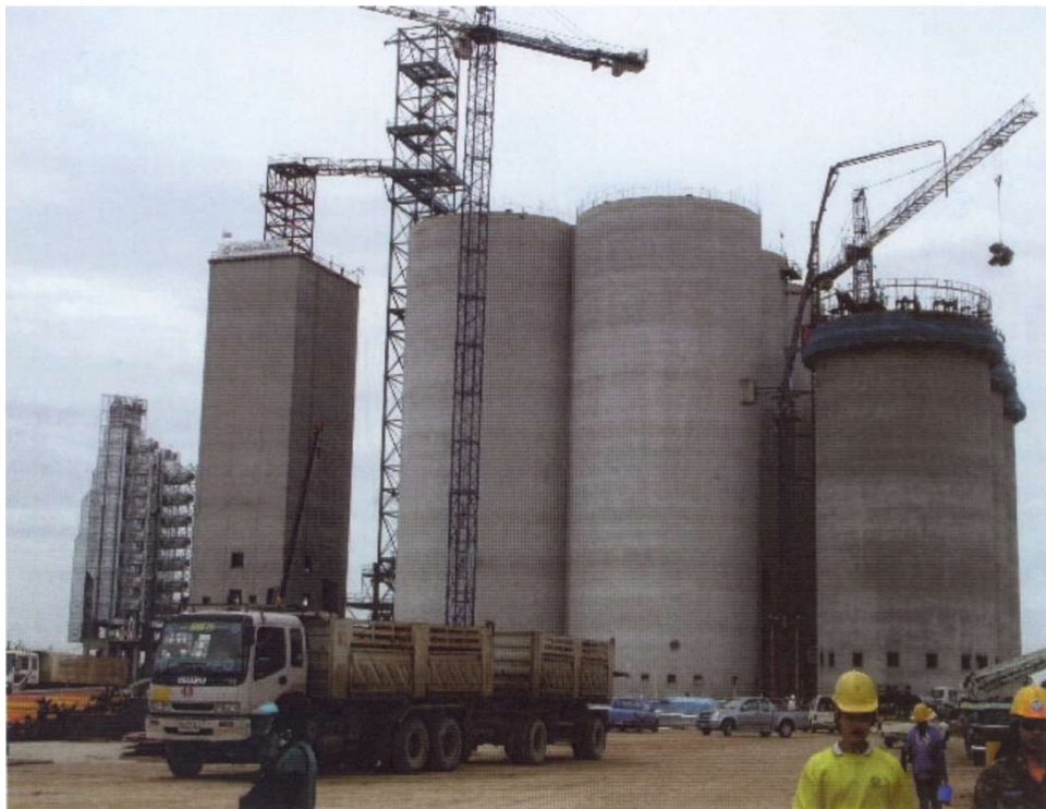
Mill & Silos Complex for CP Group, slipform in progress
