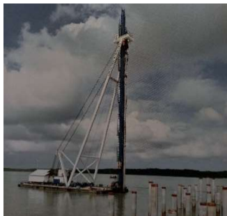
Ramlift VIII ready to drive a concrete pile
