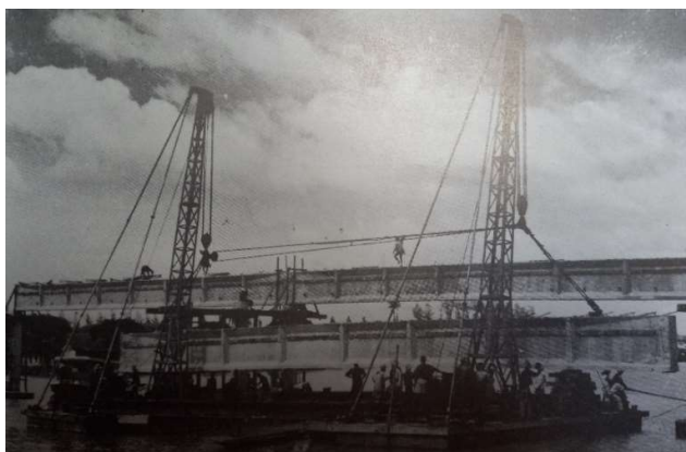
Bang Pakong River Bridge, placing of 42 ton main girder
